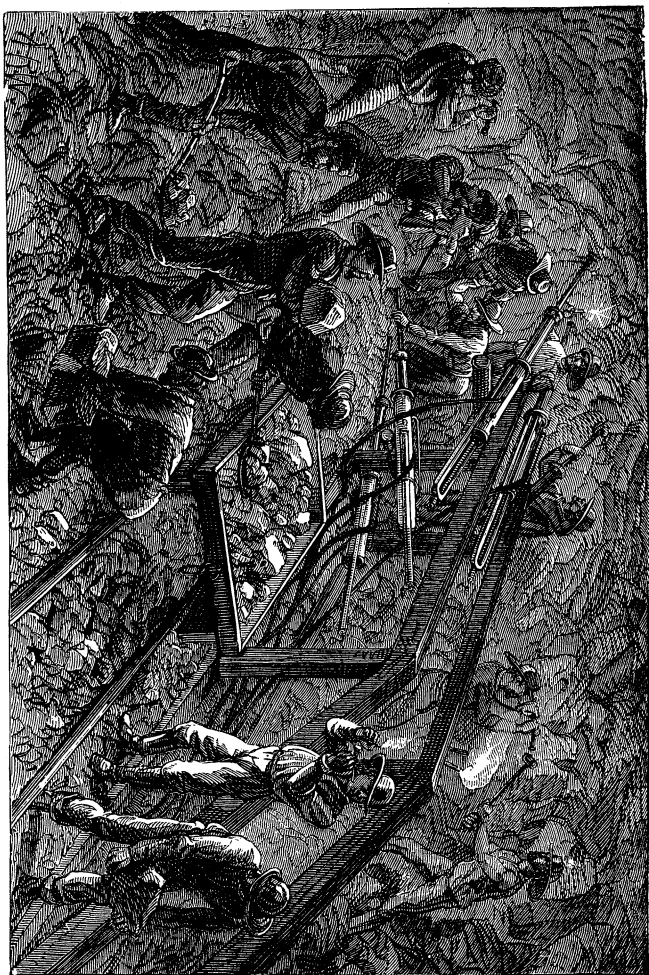
WORK AT THE HEADING IN HOOSAC TUNNEL.
