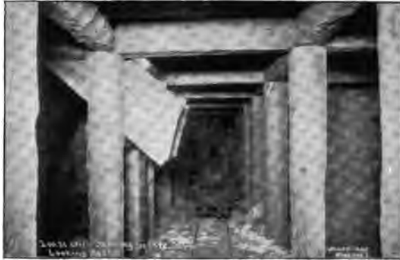
Square-Sets, Gold Coin Mine, Cripple Creek, Colorado.
