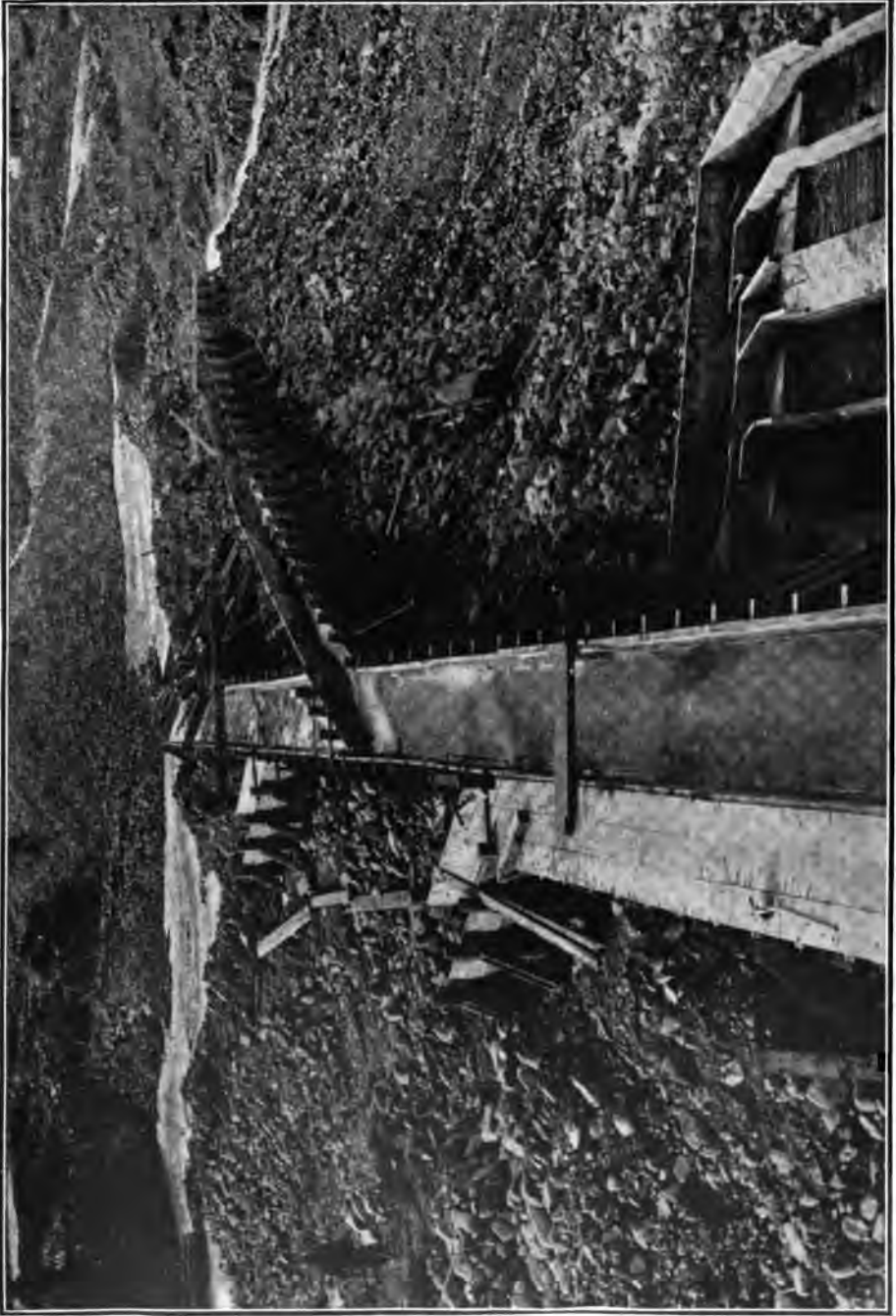
Arrangement of Sluices, Discharge End, in Hydraulic Mining. (From Engineering and Mining Journal.)
